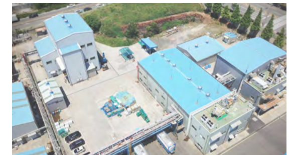
Under construction of a PO3G facility
