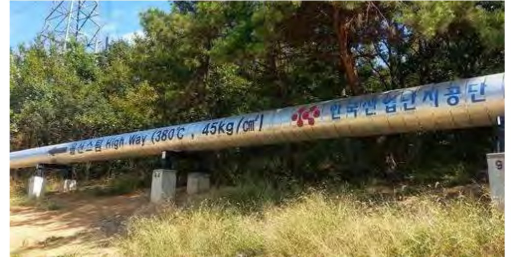
Ulsan Steam Highway supplies surplus steam between companies as part of the "Eco-Industrial Park Construction Project"
